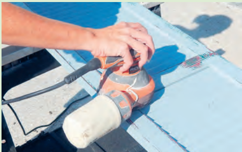
Take an electric sander and prep the shutters for some new paint.
