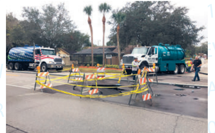
On Thanksgiving Day, a large hole literally stopped traffic on Natures Way. This was the second pipe issue to occur in the same area; the other pipe repair took place in April. Both issues occurred due to pipe collapses in the sewer drain lines. This month, the temporary repair on the second collapse will be reopened and a permanent fix installed.
