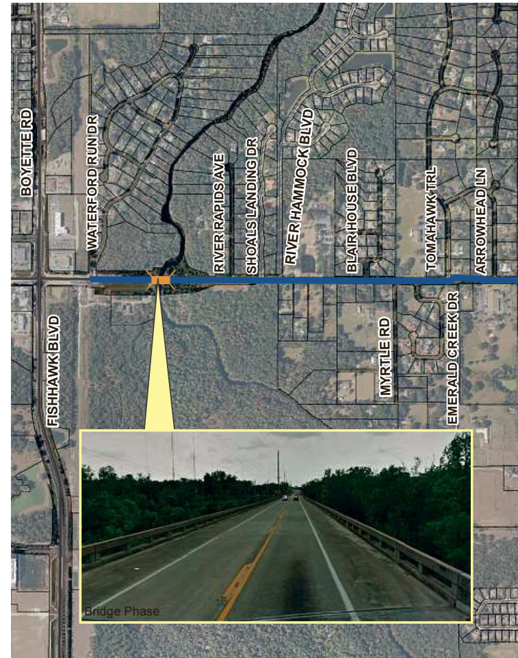
Phase One of the Bell Shoals widening project is the complete overhaul of the bridge north of the Bell Shoals-Boyette intersection.
