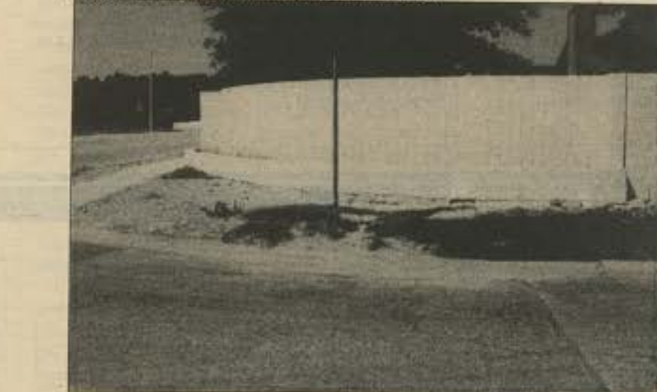
This entrance is part of the catchup the STD is still doing.
