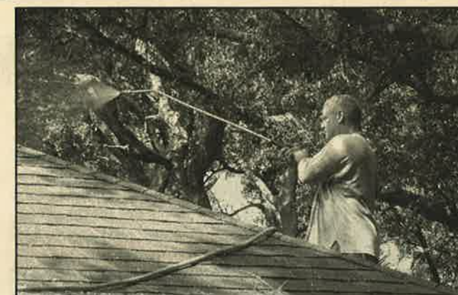
Chris Tucker, 1972 Brandon High School graduate and owner of Apple Roof Cleaning, uses chemical cleaners and mildewcide to remove and inhibit black algae growth. Tucker can be reached at (813) 655-8777.
