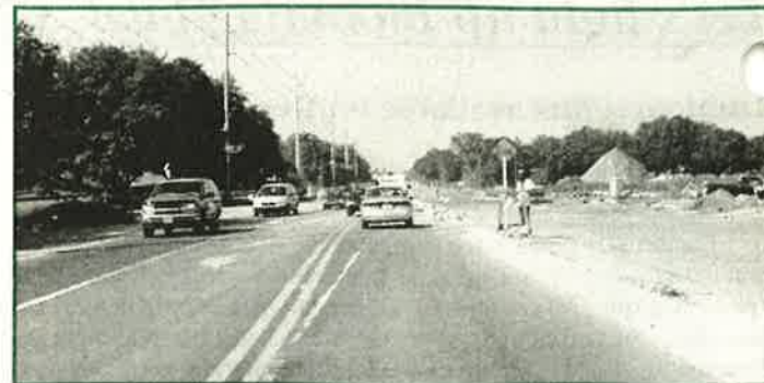
Progress continues on Bloomingdale Avenue
