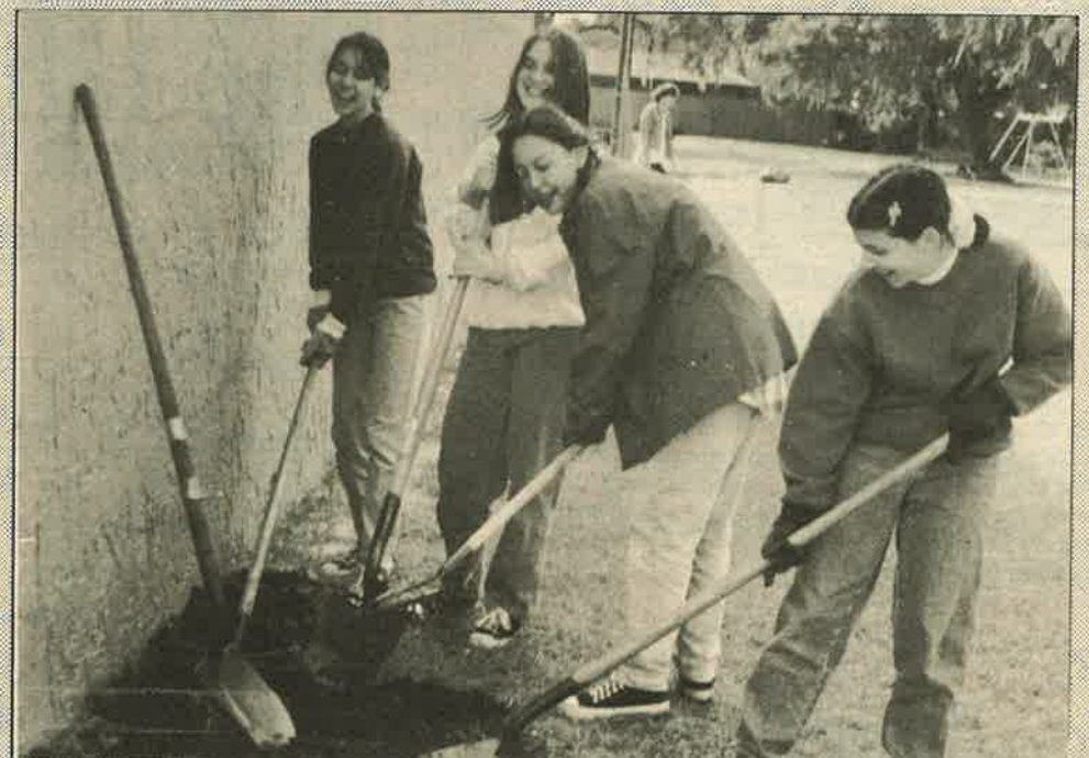
Carrie, Jessica, Nikki, and Jennifer made sure all the holes were properly filled.
