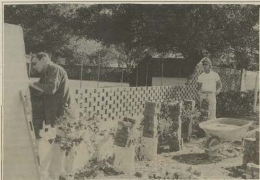
Workmen from Central Florida Landscaping repair the brickwall at Bell Shoals and Greenhollow road after it was knocked down on New Year's Eve.
