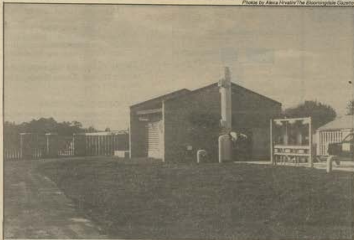
This computerized station (above) will be the only reminder of the unsightly tanks (below) and pungent odor after the tanks have been totally removed. This station is fully operational and has taken over the job of diverting the wastewater to the Valrico plant.
