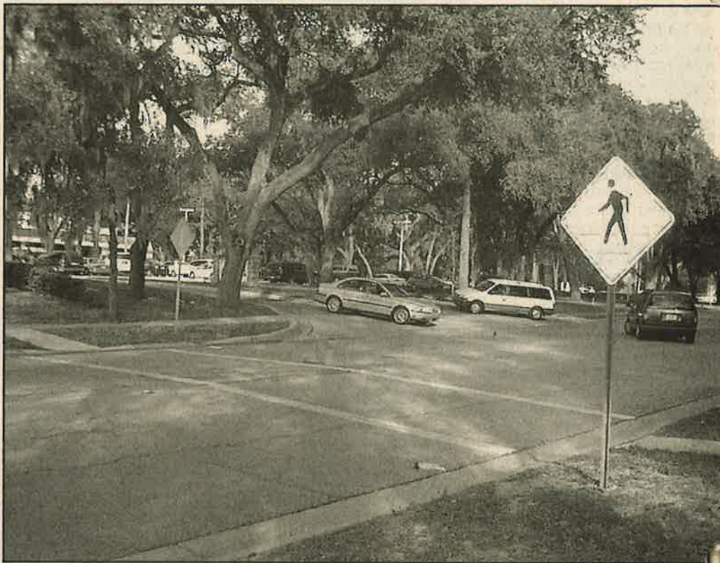
The new enhanced crosswalk on Culbreath Road between the YMCA and Bloomingdale Little League will include special strobe lights and flashers as well as a bridge across the ditch by the park. All pedestrians will be encouraged to use the crosswalk to get across safely.
