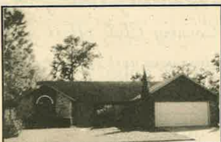
1005 Cameo Crest-Bloomingdale East High Ceilings, Lots of Sq. Footage, Sprinkler System & More!
