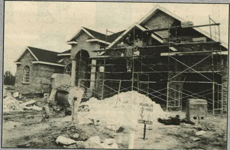
The first home nearing completion is in Ken Franklin's Cambridge Cove.
