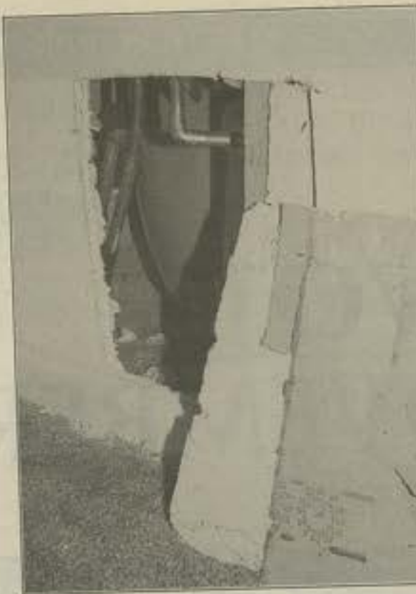
These file photos taken three years ago are still indicative of the types of problems residents are facing in homes over 18 months old. On the left, leaks are developing in walls and necessitating cutting holes plus, if they are upstairs, going through ceilings in some cases. On the right, many homeowners have complained about having to go through the cement to repair pipes.
