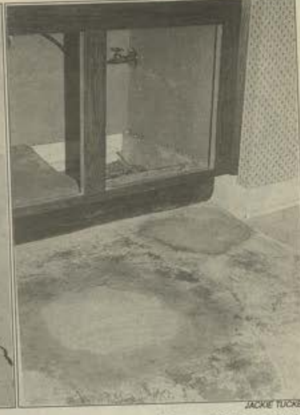
These file photos taken three years ago are still indicative of the types of problems residents are facing in homes over 18 months old. On the left, leaks are developing in walls and necessitating cutting holes plus, if they are upstairs, going through ceilings in some cases. On the right, many homeowners have complained about having to go through the cement to repair pipes.
