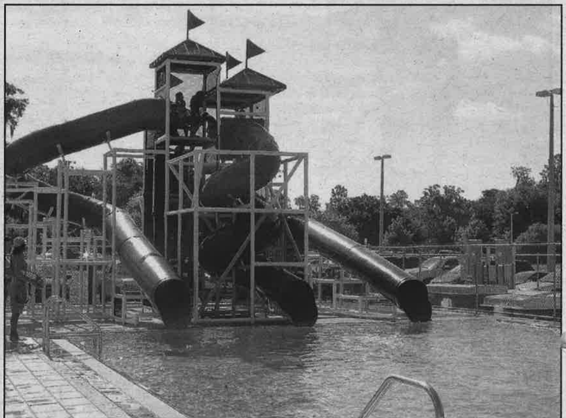
The 1,200-square-foot plunge pool features three large slides. The organization planned to open the new family fun pool and the plunge pool since it opened seven years ago. The YMCA broke ground on the project seven months ago and had the grand opening Aug. 10. The funding for the $1.5 million project came from two sources with $997,000 coming from Hillsborough County and $500,000 coming from Ray Campo. Since a large portion of the money came from the county, the pool will have community hours.
