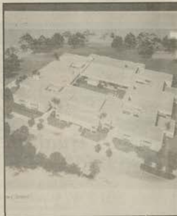
Hortense Mintz Elementary School in Heather Lakes had no access road at press time. But it is promised.
